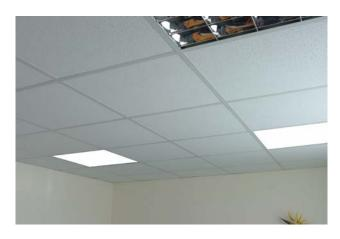
Designed to replace modular 4x 18W fluorescent trays, in suspended ceiling grid lighting, the GL-45W-HL1 LED light panel is an LED backlight module providing bright and even illumination.
